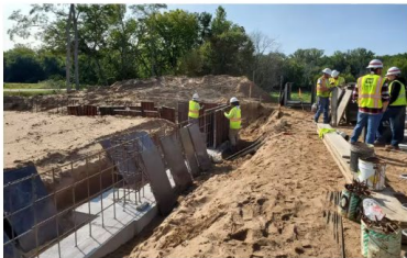
Stem wall - rebar and forms for storage building
